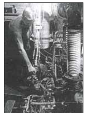
Complicated equipment keeps barges on move... 1097th mechanic knows engines inside and out
