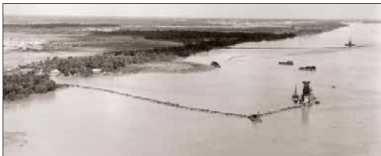
Dredge pipe line going into Dong Tam early 1967
